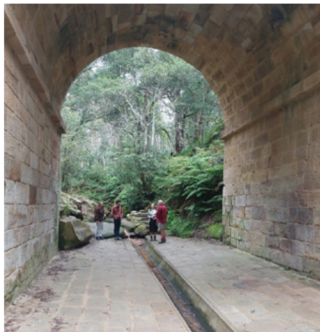
Figure 2: Lennox Bridge – Australia's oldest mainland bridge. (Photo: M McDonald)
