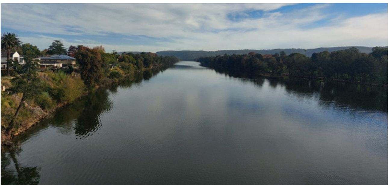
Figure 1: Nepean River Upstream of Yandii Bridge. The river is held back by the Penrith Weir elevating its 'natural' level. The edge of the Lapstone Monocline is in the distance. (Photo: M McDonald)
