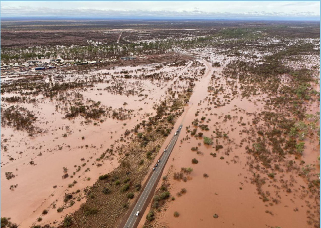
Newman Townsite (WA) & Great Northern Highway (ref Jayden Weaver - Heliwest)
