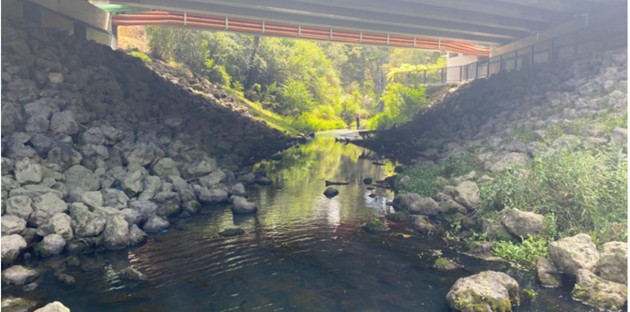
Downstream View from Weir
