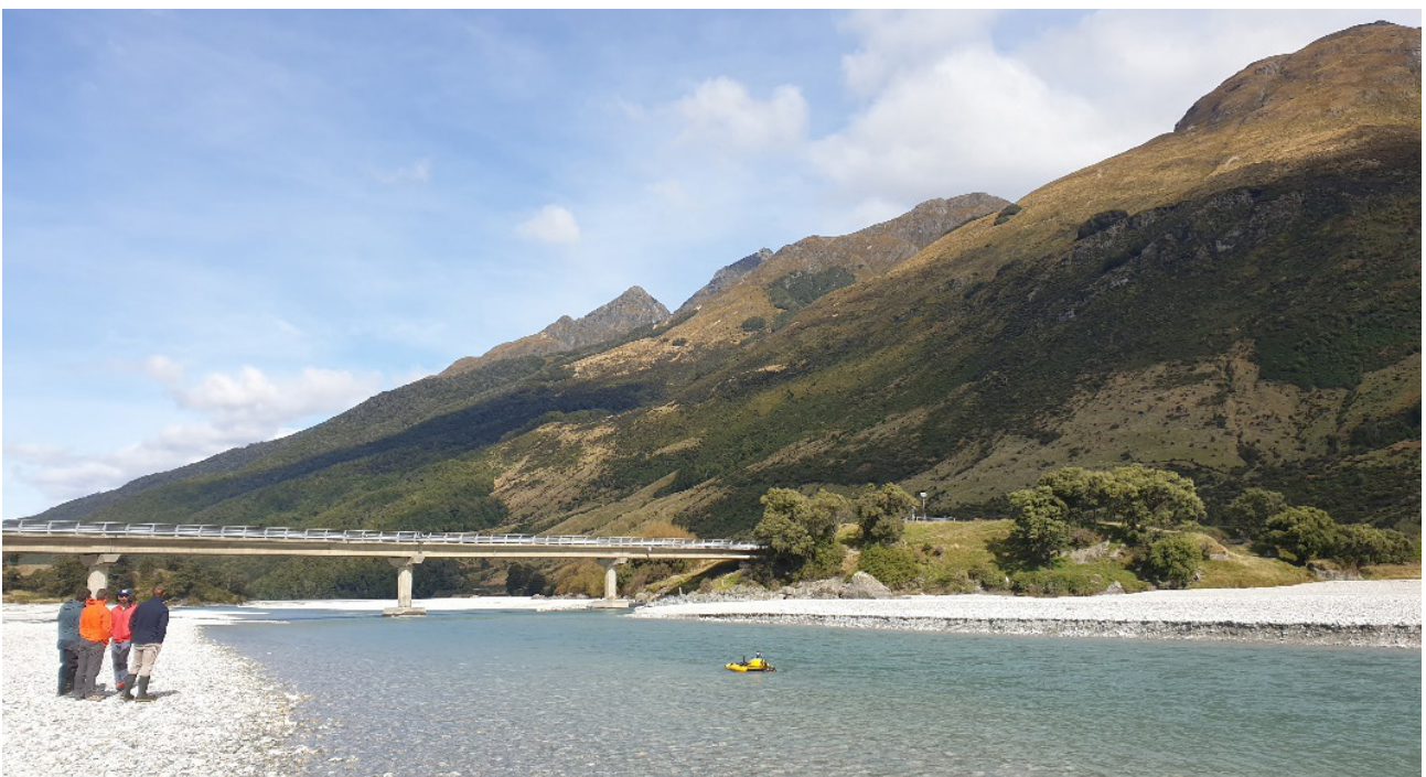
Dart River USV deployment. (The river braids, offering site selection challenges. The gauging station is located just to the right of the bridge – system solar panel is visible)
