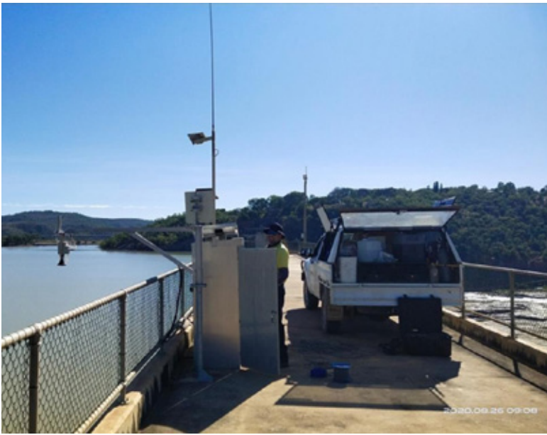
Burdekin Dam WiFi Telemetry Install Connected to Corporate Network via Satellite Broadband at Site Office
