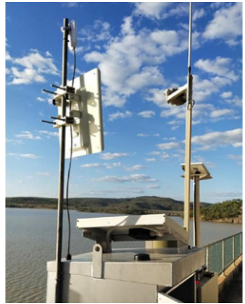
Burdekin Dam WiFi Telemetry Install Connected to Corporate Network via Satellite Broadband at Site Office
