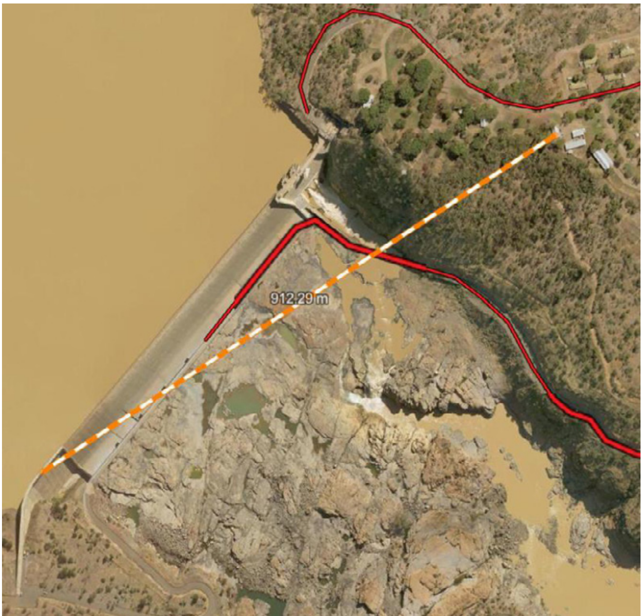
New Rookwood Weir downstream sites with no 4G reception
